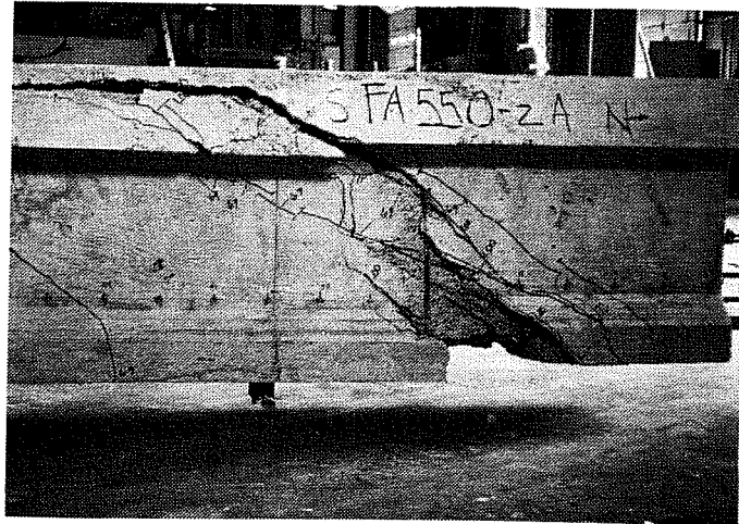
Figure 4.13 Photograph of FA550-2A Explosive Shear Failure
