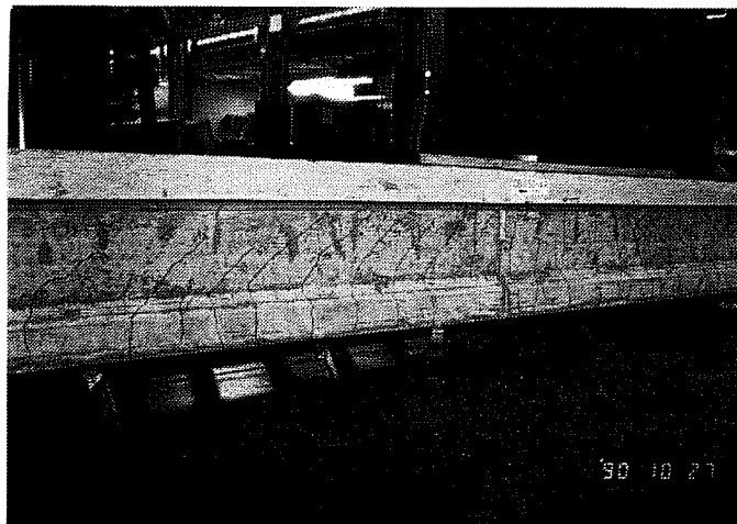
Figure 5.17 Photograph of Cracking Pattern, DB850-4A
